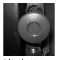
**Safety valve:** this valve acts to prevent over pressurization of the hydraulic system. If the pressure of the thermostove or plant exceeds 2.5 bar it drains the water from the circuit.
